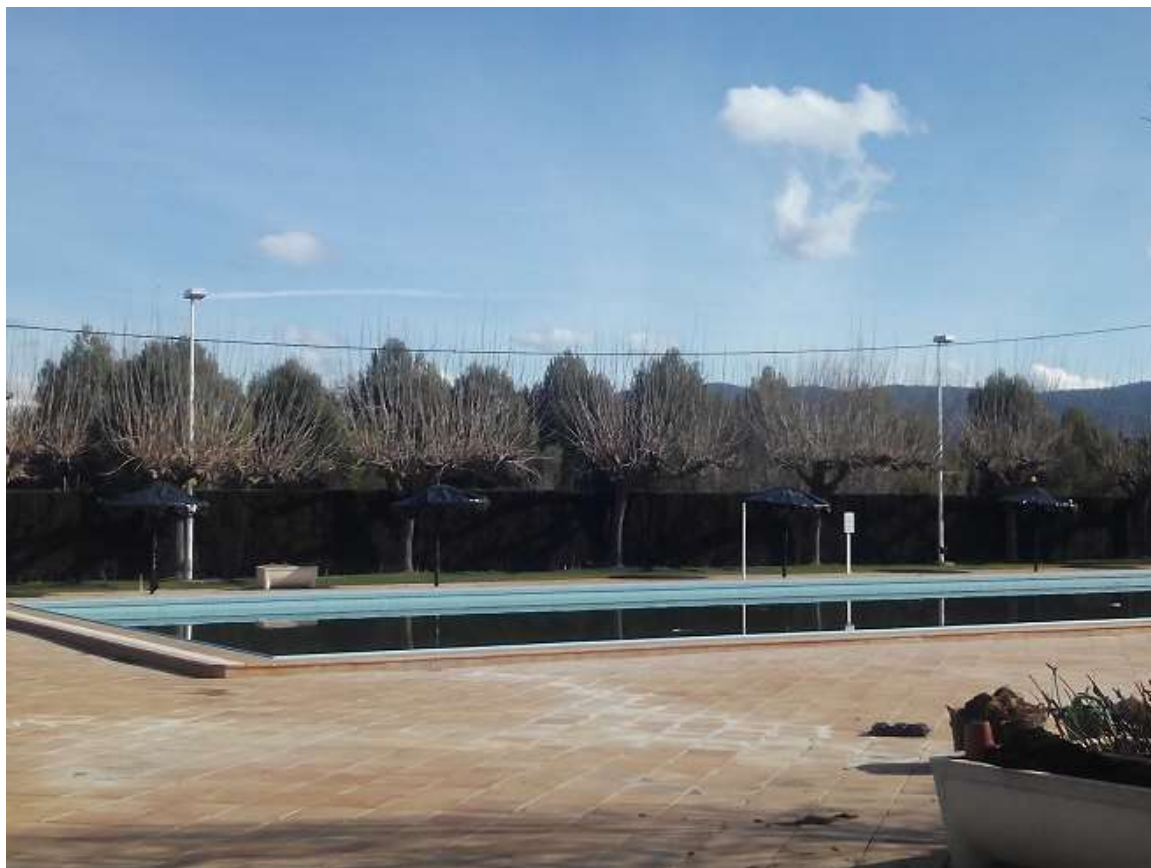
Vista general Piscina Municipal
